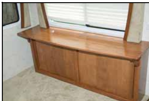
This sideboard/cabinet was installed in the dining area. The table top is taller than the sideboard to allow for storage compactness.
