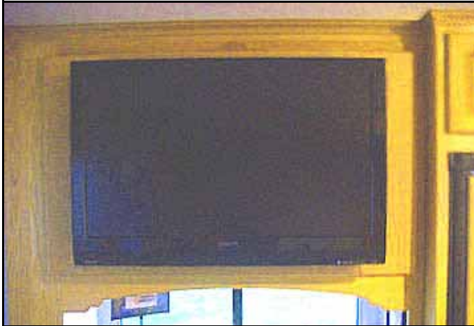
Want to install a rectangular flat screen TV in the somewhat square standard TV opening? Here's how we did it without major "deconstruction" of the existing cabinet framing.
