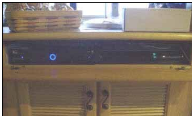
Components are mounted so that they show through the computer tray opening with the front door opened.
