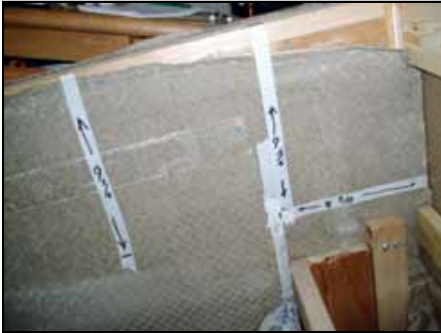
Figure 1— Do some preliminary measuring. I used masking tape to mark measurements.
