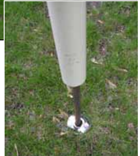
Plastic pipe drops down over metal rod and chrome ring.
