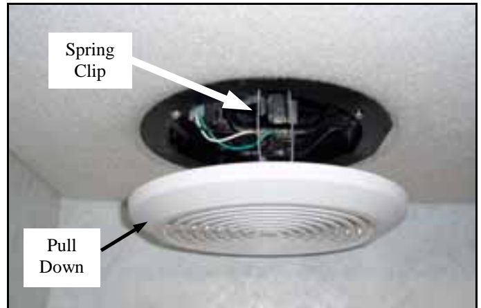
Ventline fan grill is removed by pulling down on the grill and releasing the spring tabs.
